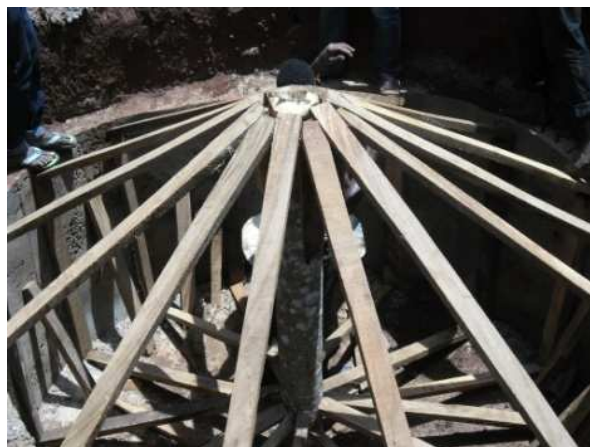
Figure 3. Gas Dome Work
