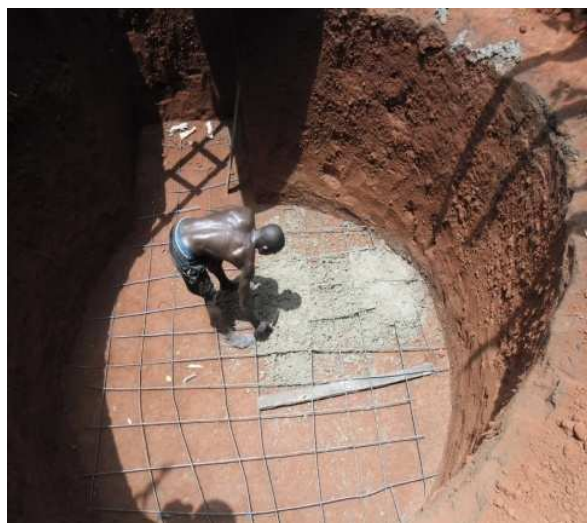
Figure 1. Excavated Pit Showing Basement Reinforcement
