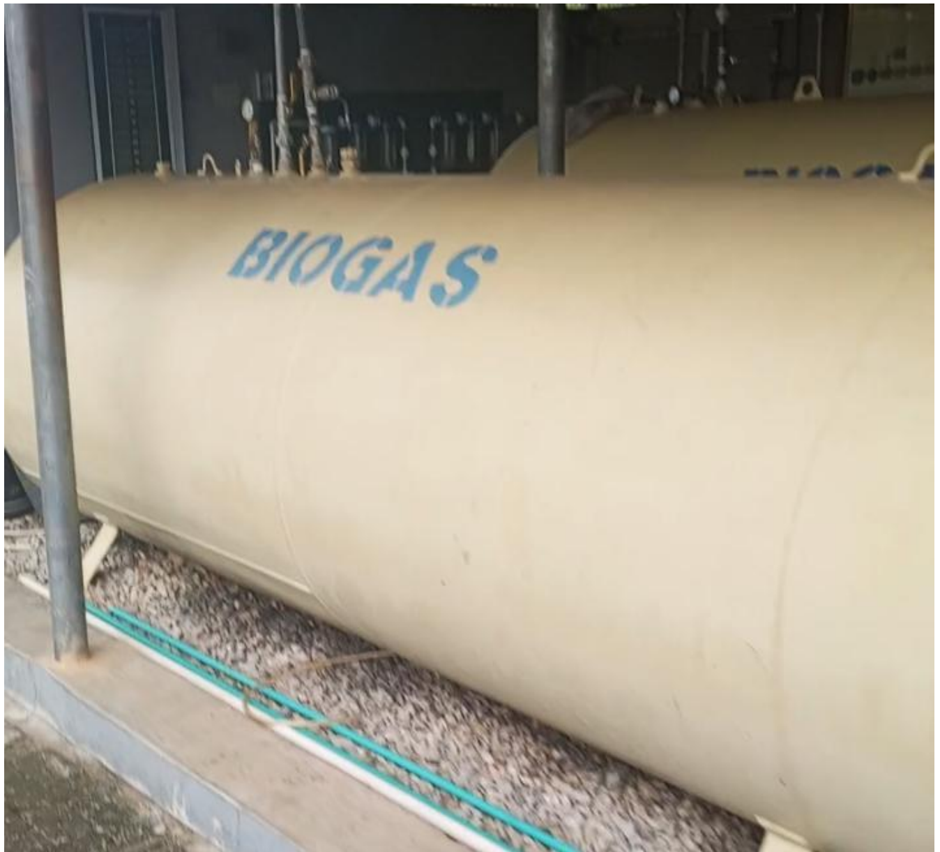
REFILLABLE COMPRESSED BIOGAS INSTALLED AT IITA SERVING THE CAMPUS KITCHEN AND OTHER RESIDENTS AND STAFF
